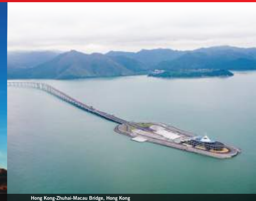
Hong Kong-Zhuhai-Macau Bridge, Hong Kong
